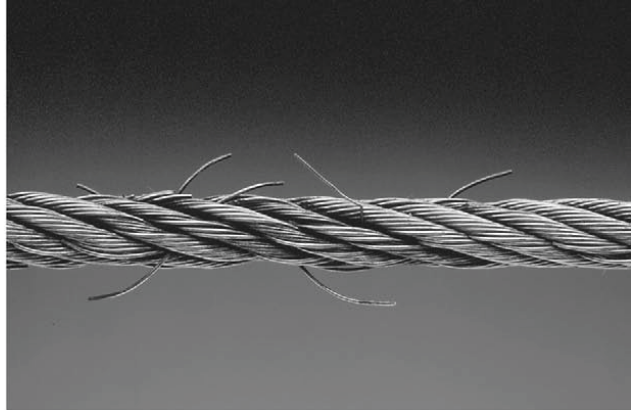
Cable With Broken Wires
